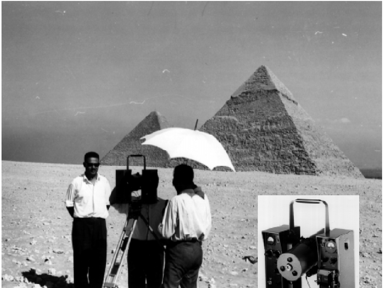
Geodimeter Model 6 in front of the Pyramids in Giza. A control measurement of the 4700-year old Cheops pyramid showed that the north side measured 231.434 m and the east side 231.379 m - a difference of only 5.5 cm from a perfect square!
